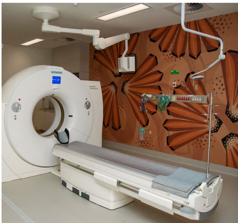
Figure 1 Example of a medical services panel in a CT imaging room
