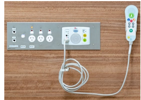
Figure 51 Example of a medical services panel with integral data outlets
