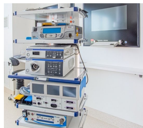
Figure 97 Example of medical services pendant configured with shelves for medical equipment in an operating room
