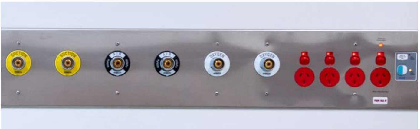
Figure 7 Example of services (connections/terminal outlets, switches and buttons) on a medical services panel
