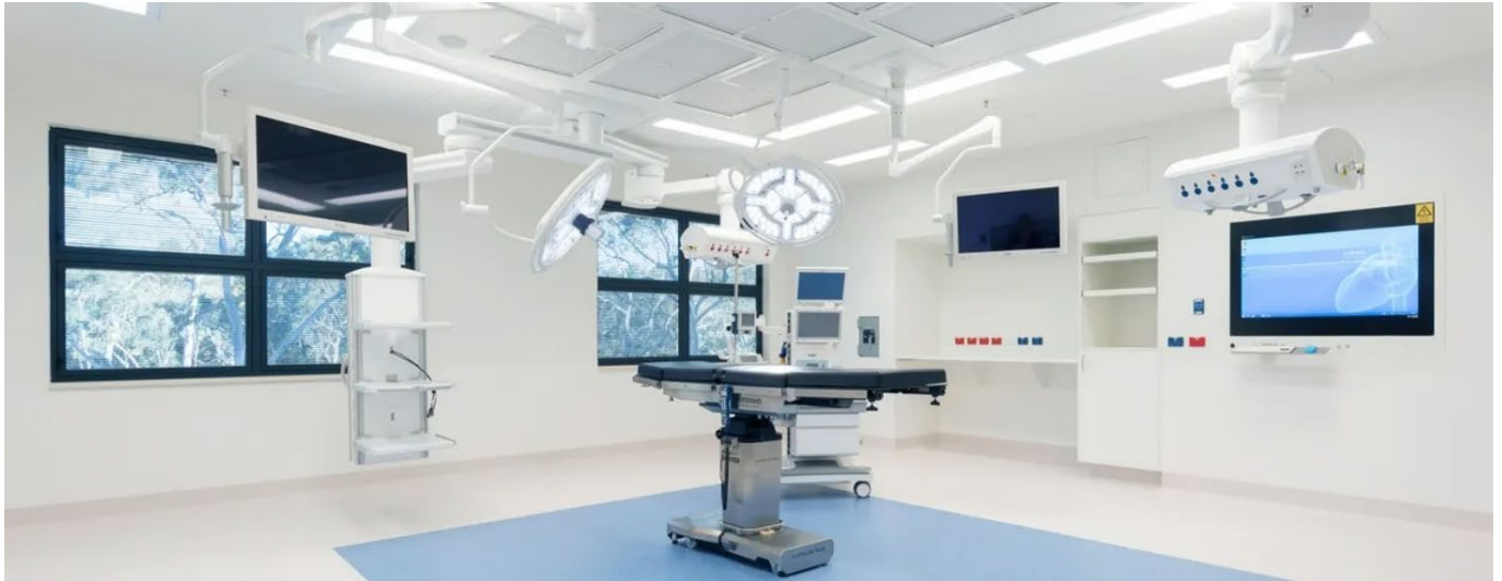
Figure 21 Example of DOR equipment (camera integral to operating light, two pendant mounted display screens and a wall mounted display screen), a 1-arm medical services pendant with horizontal services head (right) and a 2-arm medical services pendant with one horizontal services head and one vertical services head with three shelves for medical equipment (left)
