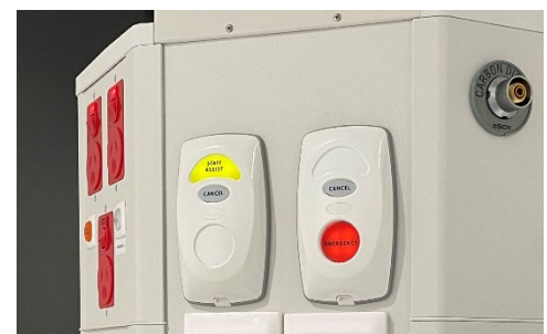
Figure 68 Example of a medical services pendant with surface mounted nurse call buttons
