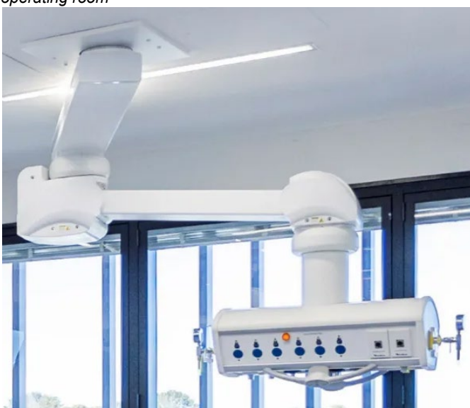
Figure 13 Example of services outlets (medical gases, power and data) and services accessories (suction adapters) on a horizontal services head in an operating room
