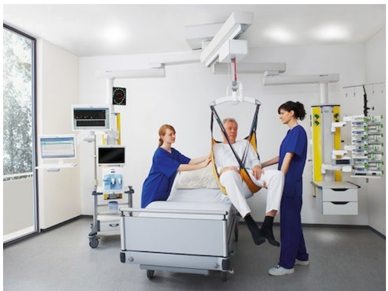
Figure 125 Example of a 3-arm pendant with two service heads and a patient lifter
