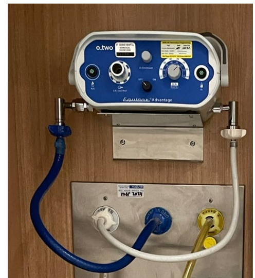
Figure 31 Oxygen and nitrous oxide blender
