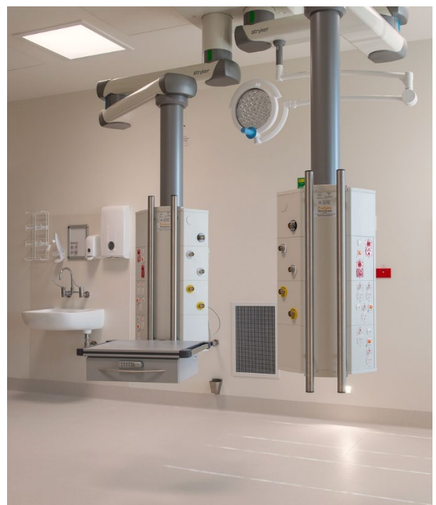
Figure 2 Example of medical services pendants in an intensive care bedroom
