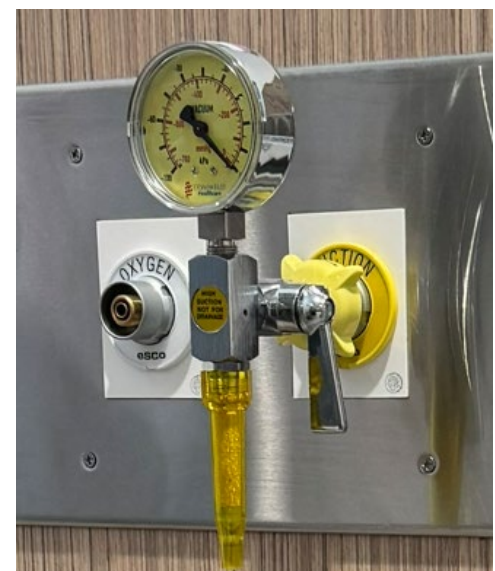
Figure 27 Example of a suction Adapter
