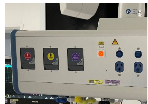
Figure 67 Example of a medical services pendant with flush nurse call buttons
