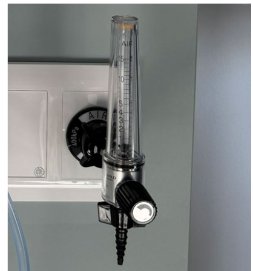
Figure 29 Example of a medical air flowmeter
