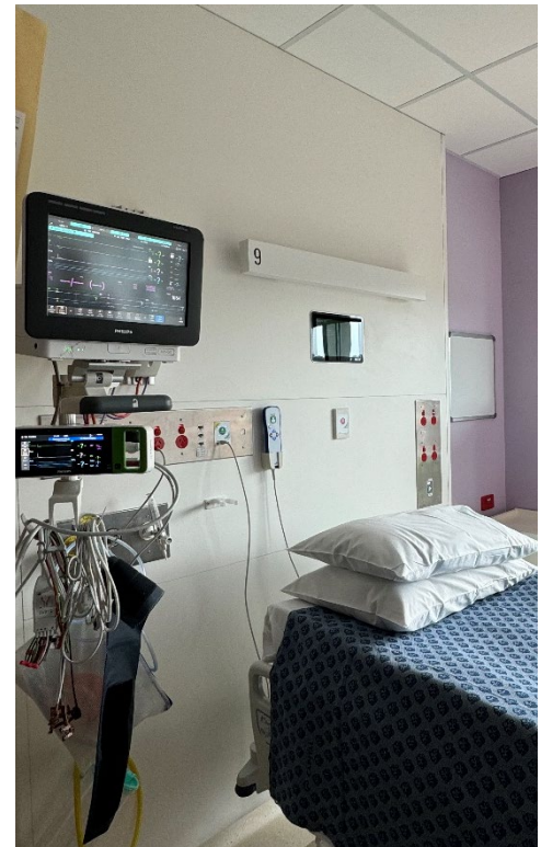
Figure 108 Example of a double-row medical services panel layout (to clinical side/patient's right) and a multi-row/vertical medical services panel (to patient/visitor side) in an inpatient bedroom
