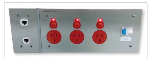
Figure 104 Example of a modular medical services panel with one module for data and another for electrical outlets
