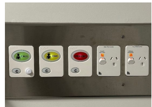
Figure 66 Example of a medical services panel with flush nurse call buttons
