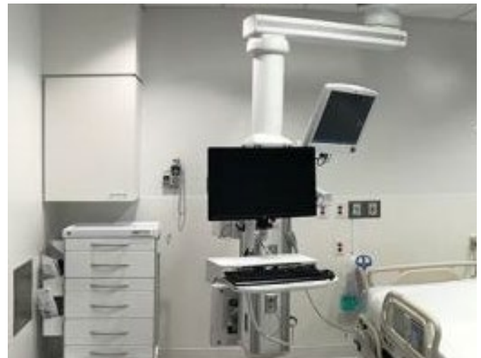
Figure 18 Example of a display screen and a keyboard on a drawer shelf mounted directly on a vertical services head
