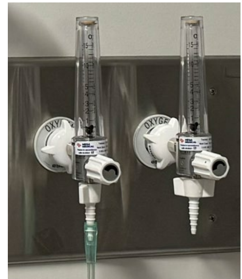
Figure 26 Example of oxygen flowmeters
