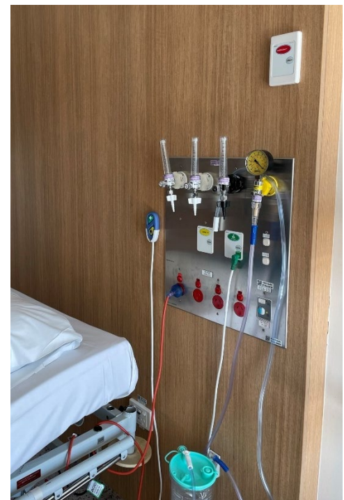
Figure 109 Example of a multi-row medical services panel layout to a patient bay
