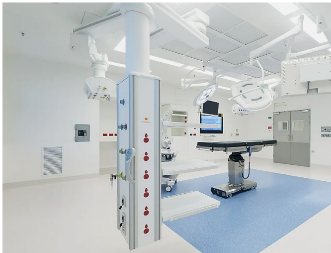
Figure 17 Example of services outlets (medical gas, power, audio-visual, and communications outlets), services head accessories (shelves) on a vertical services head in an operating room
