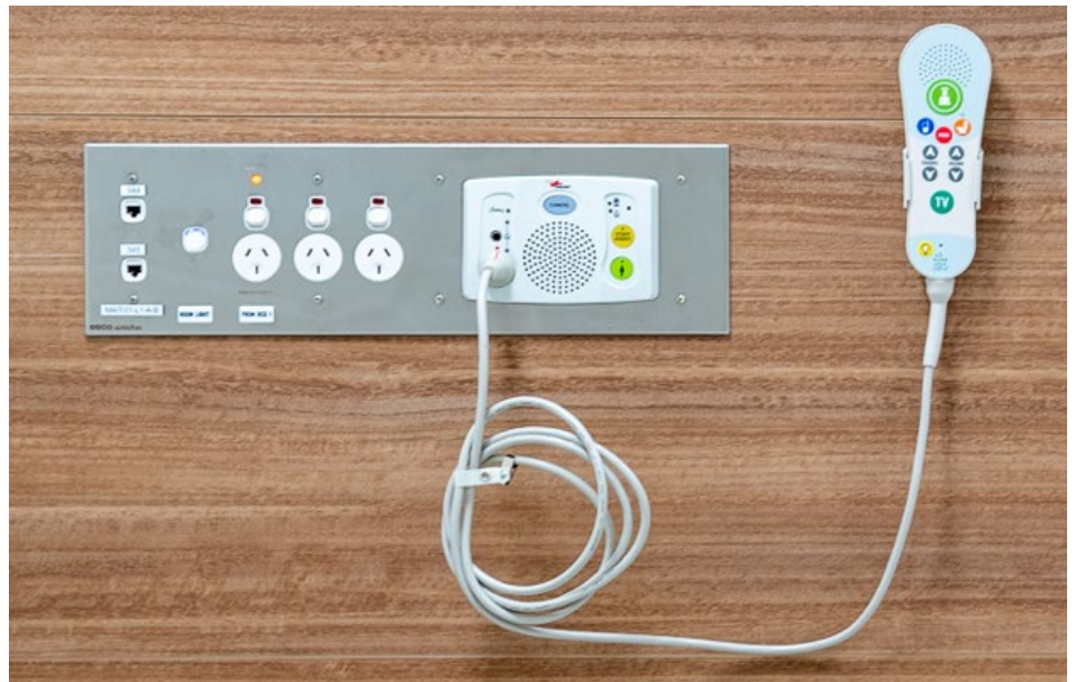
Figure 70 Example of a medical services panel with a combined patient to staff call, staff assist call, patient call handset connection and speaker
