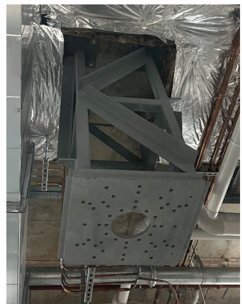
Figure 119 Example of a structural mounting frame (cotton reel) secured to a concrete slab for installation of a medical services pendant
