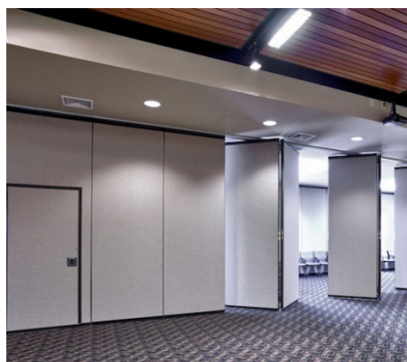
Figure 19 Example of operable wall with an inset door to one panel
