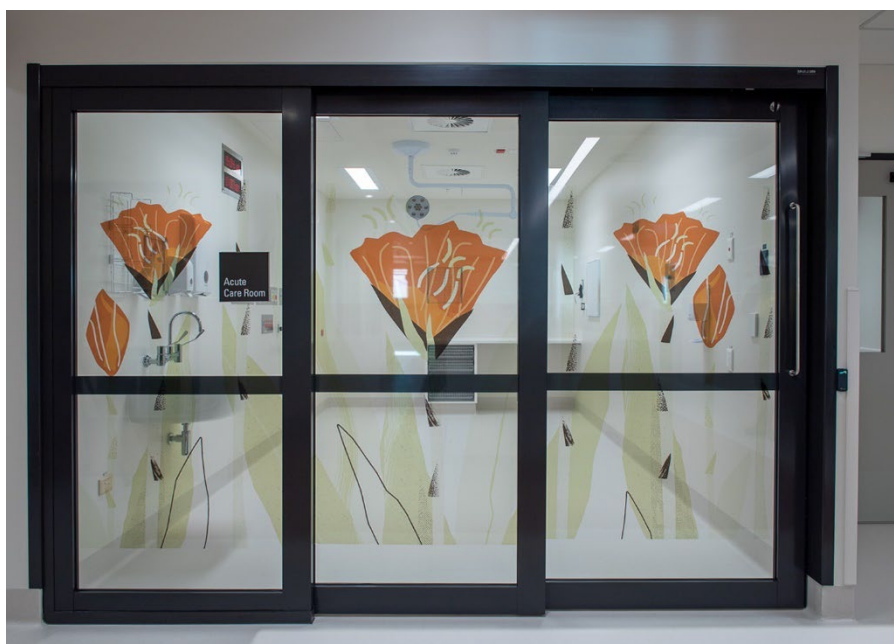
Figure 67 Example of glazing decal to fully glazed stacking door for an acute care room
