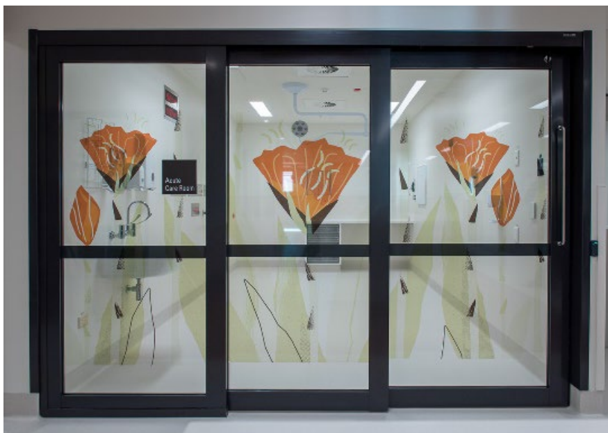
Figure 12 Example of manually operated stacking door with two leaves stacking behind a fixed panel to an acute care room
