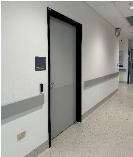
Figure 25 Example of single leaf solid core door
