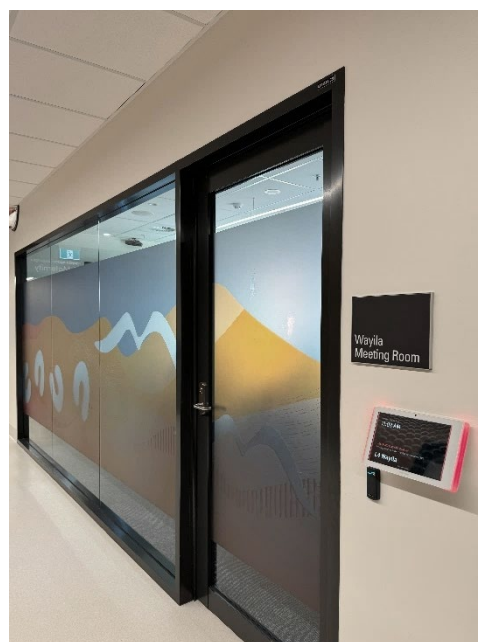
Figure 68 Example of glazing decal to a fully glazed door and associated glazing
