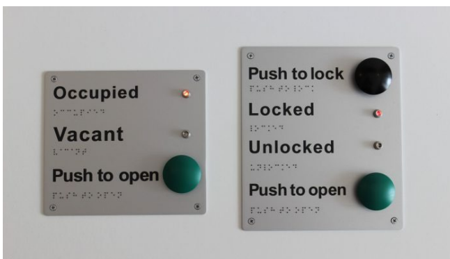
Figure 59 Example of push to open and push to lock buttons of a privacy system for accessible toilets and parenting rooms
