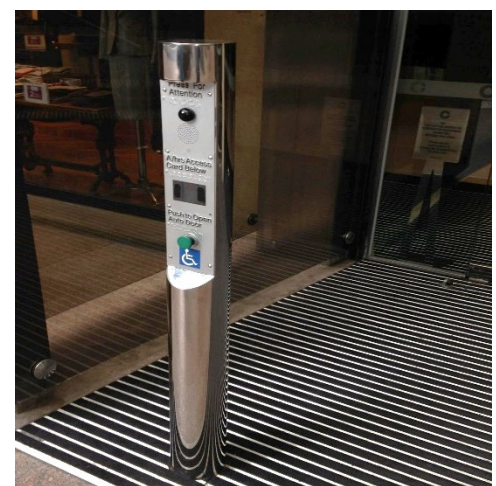
Figure 83 Example of door controls (swipe card for after hours and push to open button) and intercom on bollard
