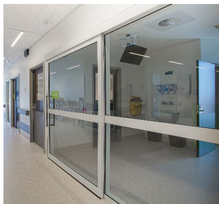
Figure 29 Example of a fully glazed, framed door with mid-rail
