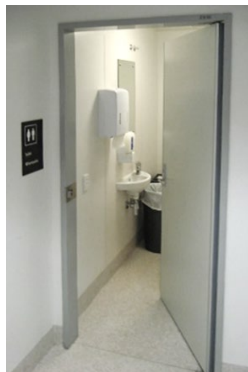
Figure 10 Example of pivot door to toilet with emergency release hardware
