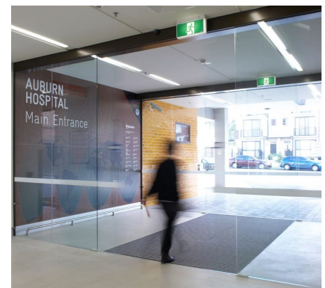
Figure 30 Example of a fully glazed, frameless automatic sliding door
