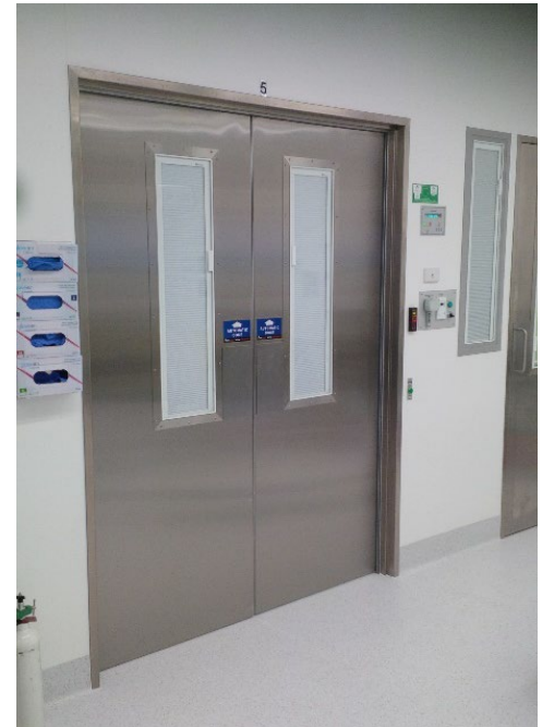
Figure 38 Example of double doors containing vision panels with integral blinds
