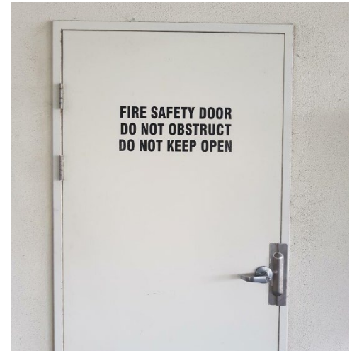
Figure 48 Example of fire door with statutory signage
