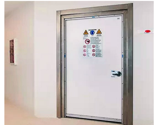
Figure 46 Example of RF shielding door to MRI room
