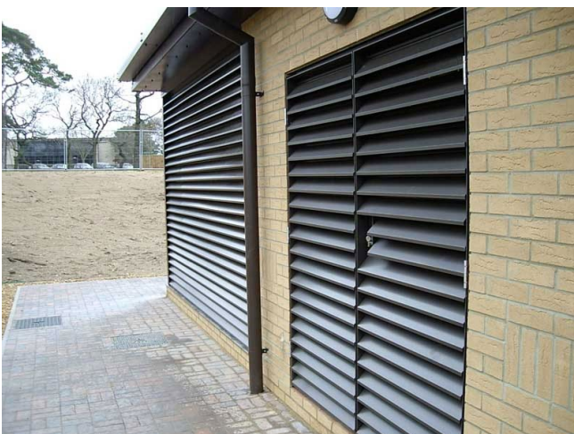
Figure 51 Example of external acoustic louvred door to plant room
