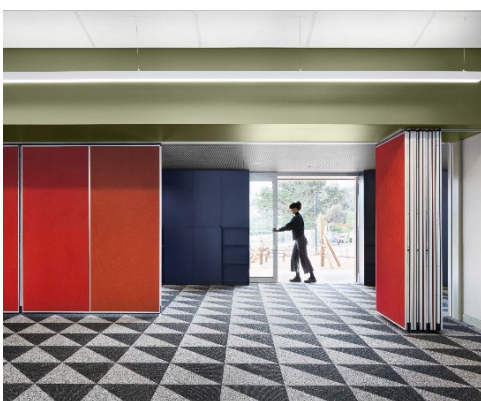
Figure 18 Example of operable wall with some panels stacked
