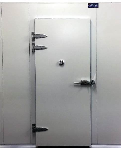
Figure 56 Example of cool room hinged door
