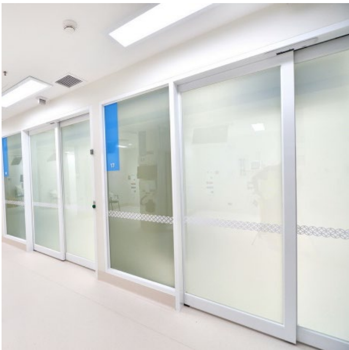
Figure 41 Switchable glass in ICU when turned off (opaque)
