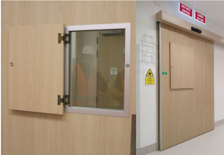
Figure 43 Example of custom hinged vision panel cover to sliding door
