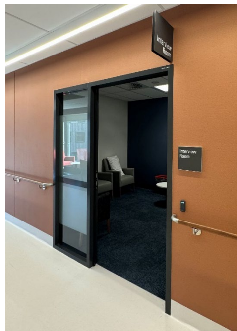
Figure 66 Example of door to interview room with sidelight finished with privacy film
