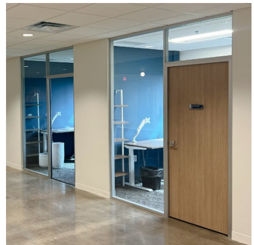
Figure 37 Example of transom window over solid core door to office
