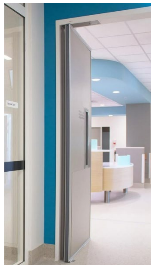
Figure 9 Example of pivot door in corridor
