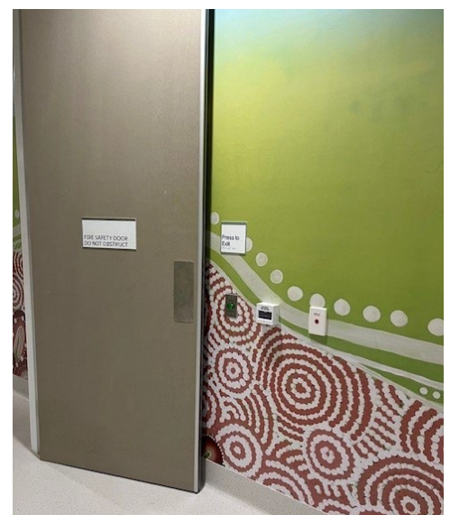
Figure 82 Example of door controls located on top of graphic design features and are therefore difficult to identify
