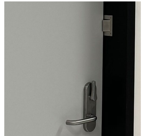
Figure 80 Example of retractable stop to a pivot door on a sanitary compartment
