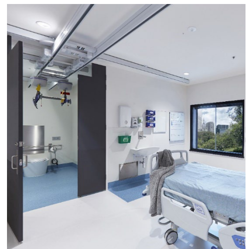
Figure 24 Patient lifting track transferring from a bariatric bedroom to the associated ensuite
