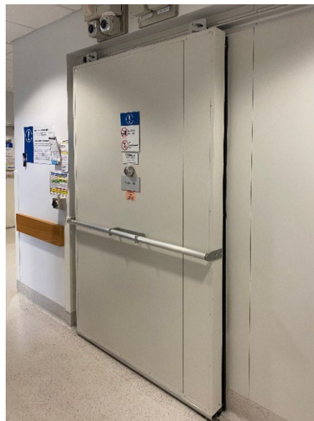
Figure 55 Example of cool room sliding door to body holding in mortuary unit
