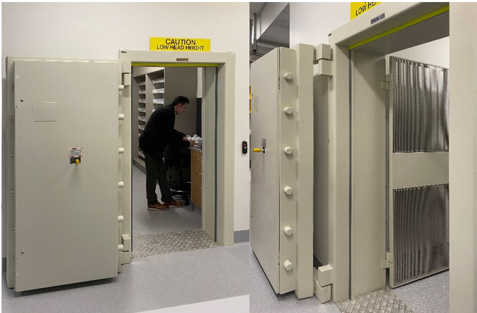
Figure 53 Example of strong room door to accountable drugs store in pharmacy
