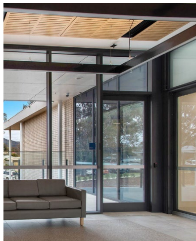
Figure 36 Example of transom window to external single door
