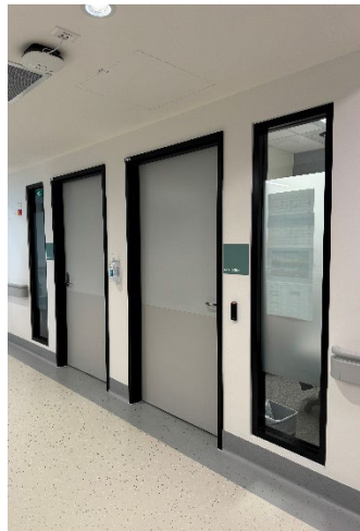
Figure 33 Example of sidelights (separate from door frame) to offices on an inpatient unit
