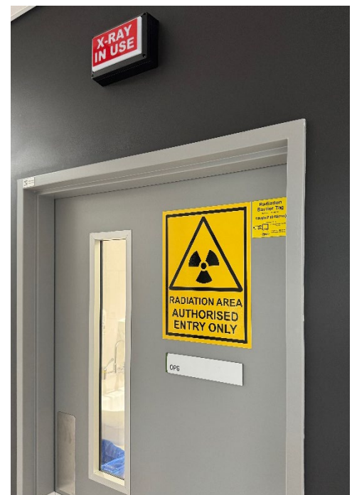
Figure 45 Example of lead lined door to OPG room with x-ray in use light above and radiation warning signage
